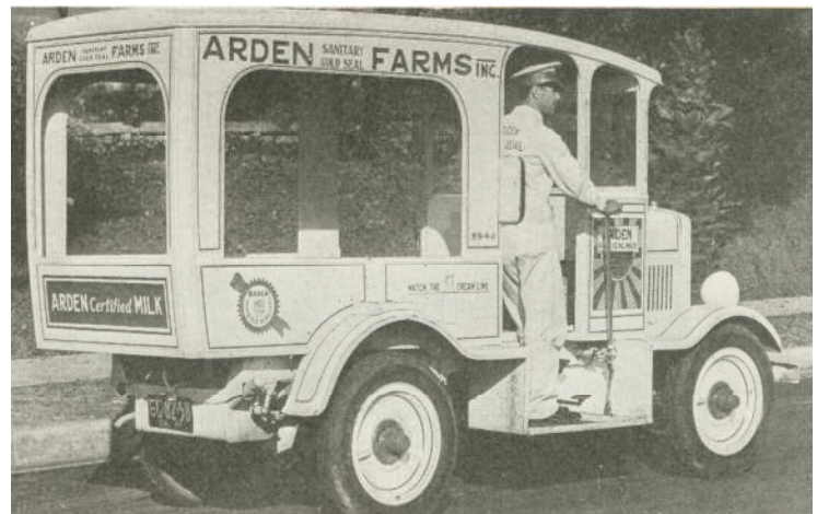
A house-to house milk delivery truck used by Western Dairy Products Inc. It is a Divco built by D etroit I ndustrial V ehicle C ompany and is equipped with a canopy express body.
